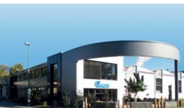
Local production plant
