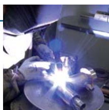
Experienced and qualified welders
