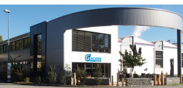
New production plant
